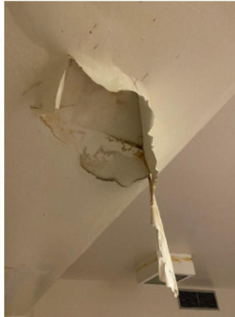
HVAC/Roof issues cause damage to interior ceiling
