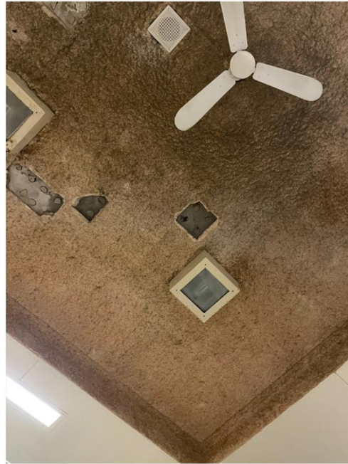
Falling Acoustic Tiles
