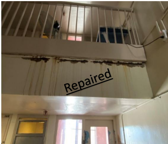
Upper tier steel railing rusted
