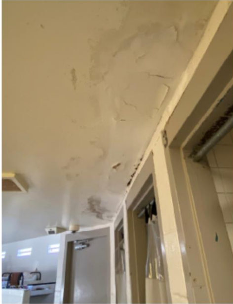
Damage from 2nd Tier Shower Leaks
