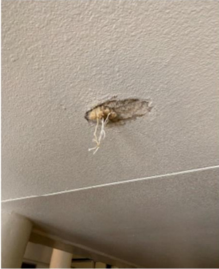
Water Damage – Ongoing Leak
